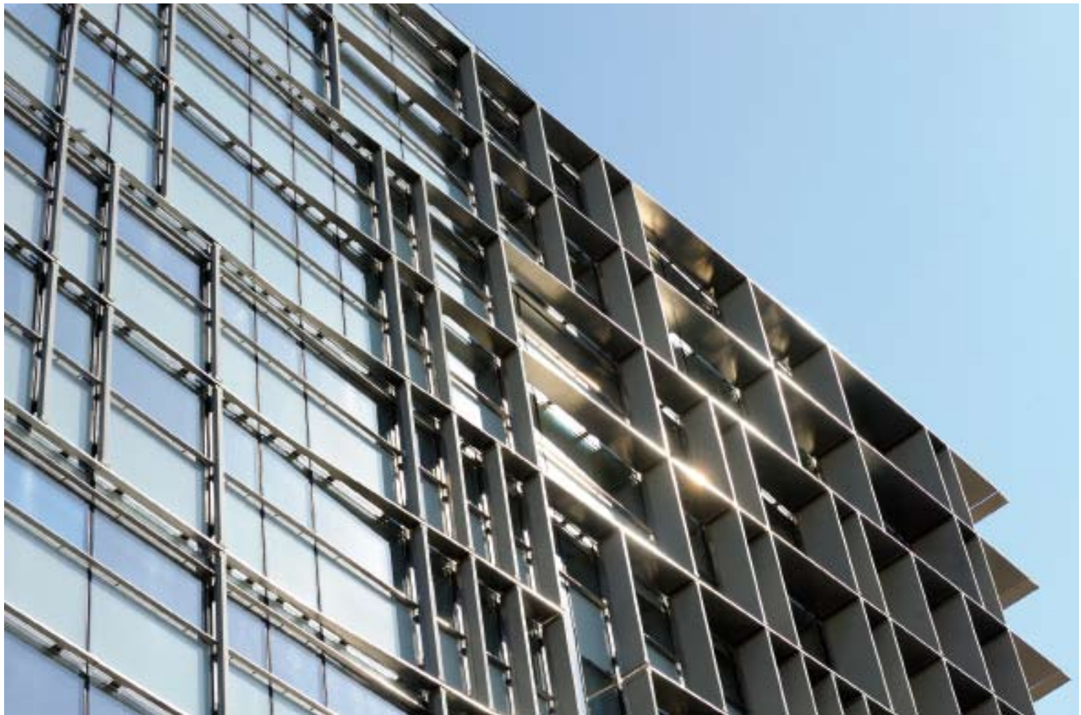
↑ | Façade detail , double skin with brushed stainless steel horizontal sun breakers and solid Pietra Serena vertical stone louvers ← | Floor plans , ground, typical, fifth floor
