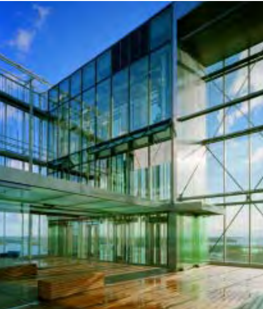
The courtyard of the Kone Building in Espoo is shielded from the wind, and enjoys a nice view out over the bays and the sea.
