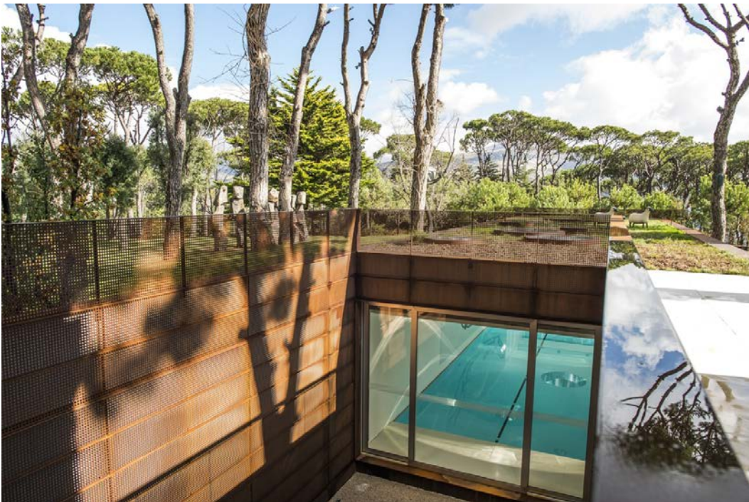
A view of the pool's sun roof. Roger Moukarzel for The Wall Street Journal
